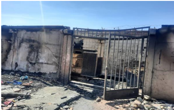
A: Transformer site reported to be the genesis of outbreak
